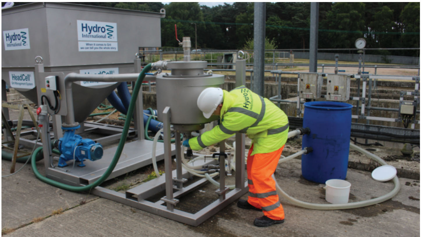
Wastewater grit sampling underway with Hydro International’s HeadCell pilot unit.
