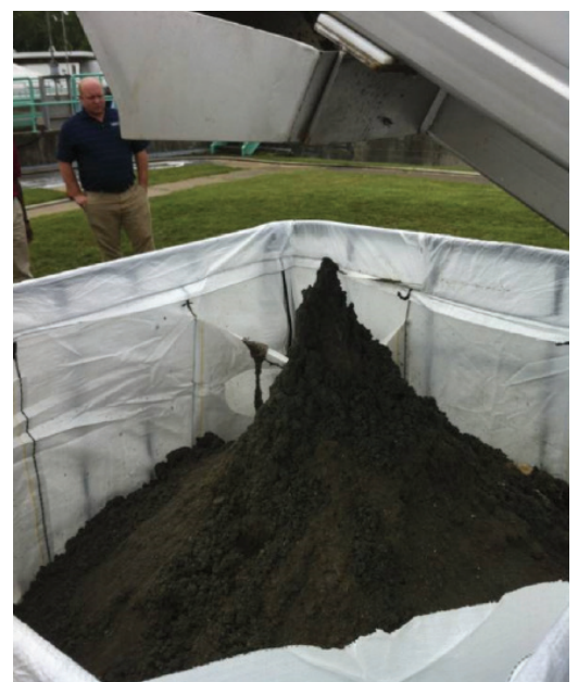
Collected grit following grit removal
